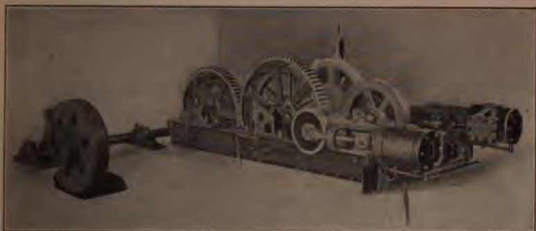
Combined Hoisting and Swinging Engine of Floating Dipper Dredge. Figure 78.
